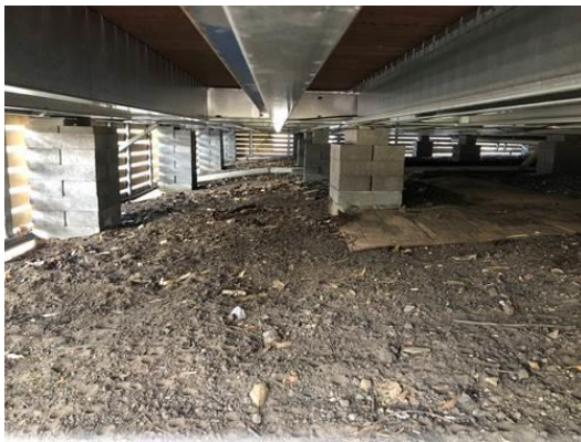
Photo 1: Example of proposed amenities building foundation - blockwork piers on compacted ground
