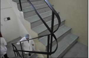
**Figure 50**. Curved steel handrails located in stairwell located between floor five and floor three.(Source: Heritage 21, 09.03.16)
